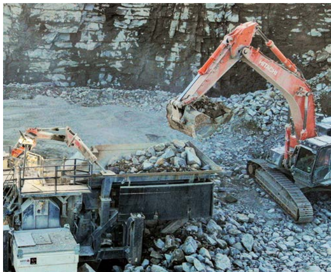
CRUSHING AND SCREENING p. 4
